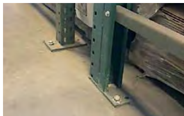
Typical low-corrosive environment — interior warehouse.
