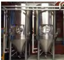
Typical high-corrosive environment — food-processing plants.
