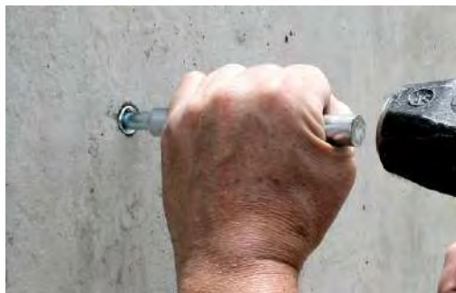
Anchor being set with hand setting tool.
