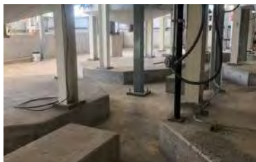
Typical medium-corrosive environment — exterior anchorage.
