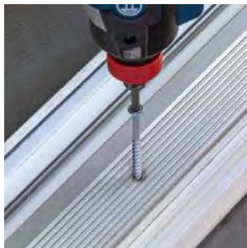
Sliding door track installation
