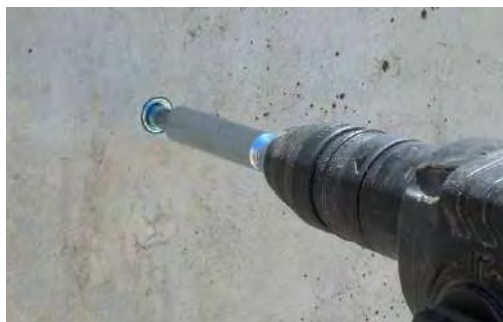
Anchor being set with SDS setting tool.
